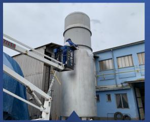
Before the commencement of the implementation, we had to prepare the beer tank for the application of thermal insulation, i.e., cover the parts that did not need insulation. Thermal insulation application for beer tanks at Pilsner Urquell. The materials used were Bronya Antikor and Bronya Classic with a thickness of 2.5mm. The issue with condensation cannot be resolved by conventional insulation because standard insulation methods are unable to prevent condensation.
